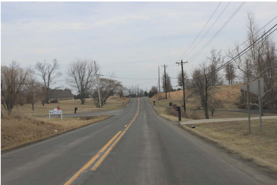
Figure 5: KY 251 at Bates Road (looking north)
